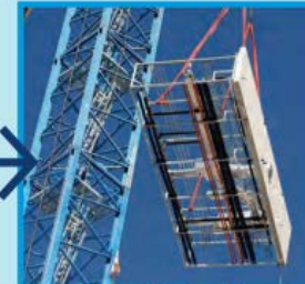
A tower crane lifting the MEP corridor racks
