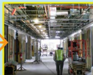
MEP corridor racks being installed
