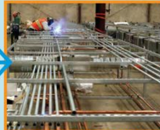
Dedicated MEP crews building the MEP corridor racks at "bench height"
