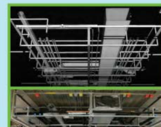
MEP corridor racks BIM model design and final MEP corridor racks installed
