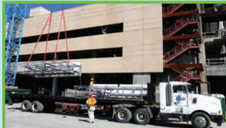
MEP corridor racks being delivered to the jobsite
